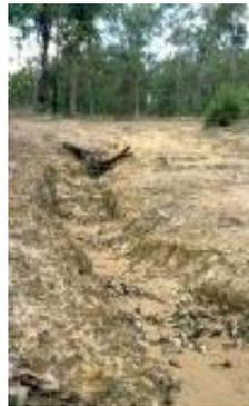
2.10 A badly eroded access track. Erosion can be avoided by post-harvest draining of all snig and haulage tracks.
